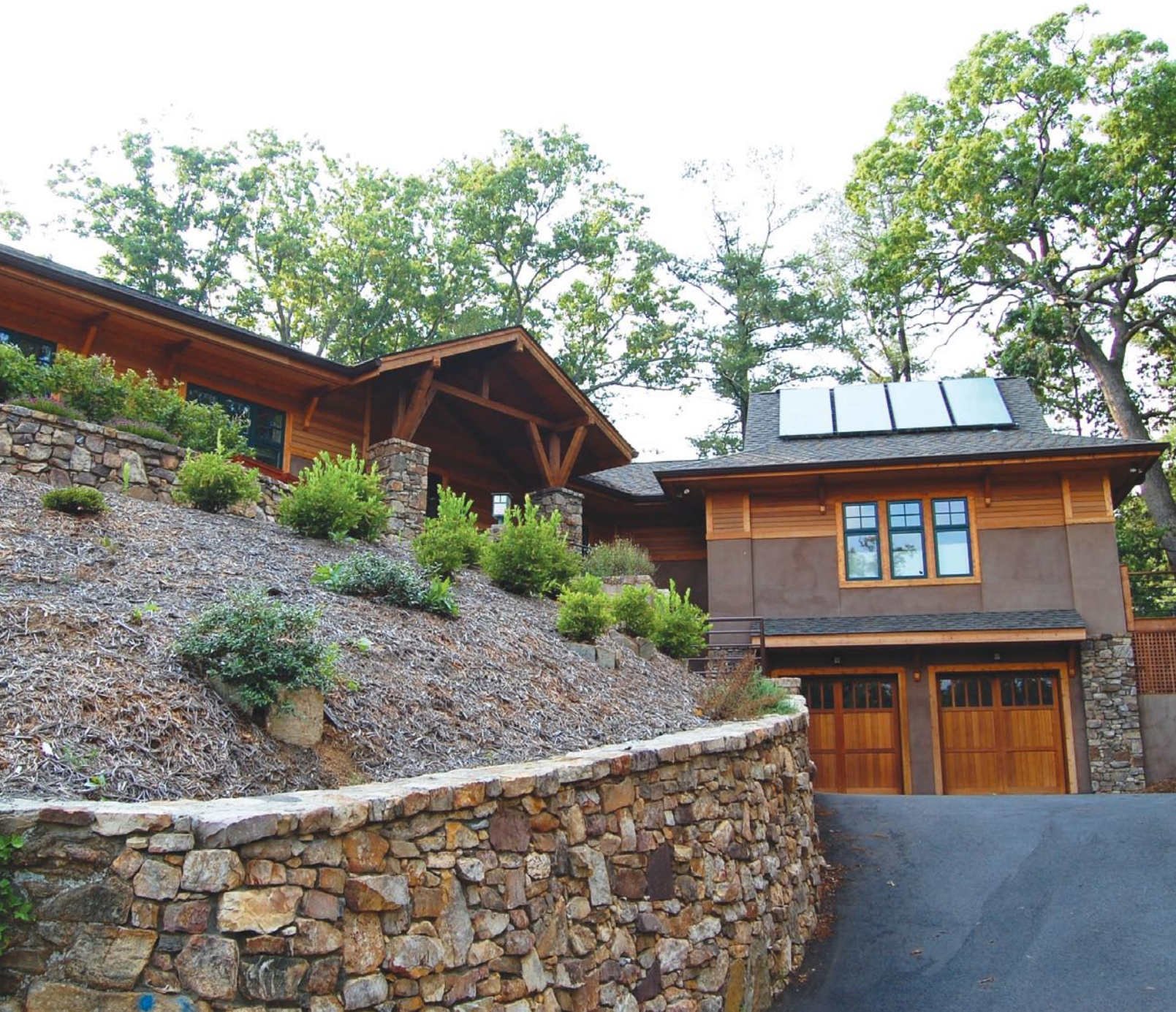
The Chapman residence has solar hot water and radiant floor heating installed by Sundance Power Systems.
